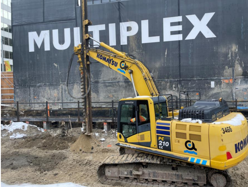
Pictured: One Delisle progress update as of March 2022
