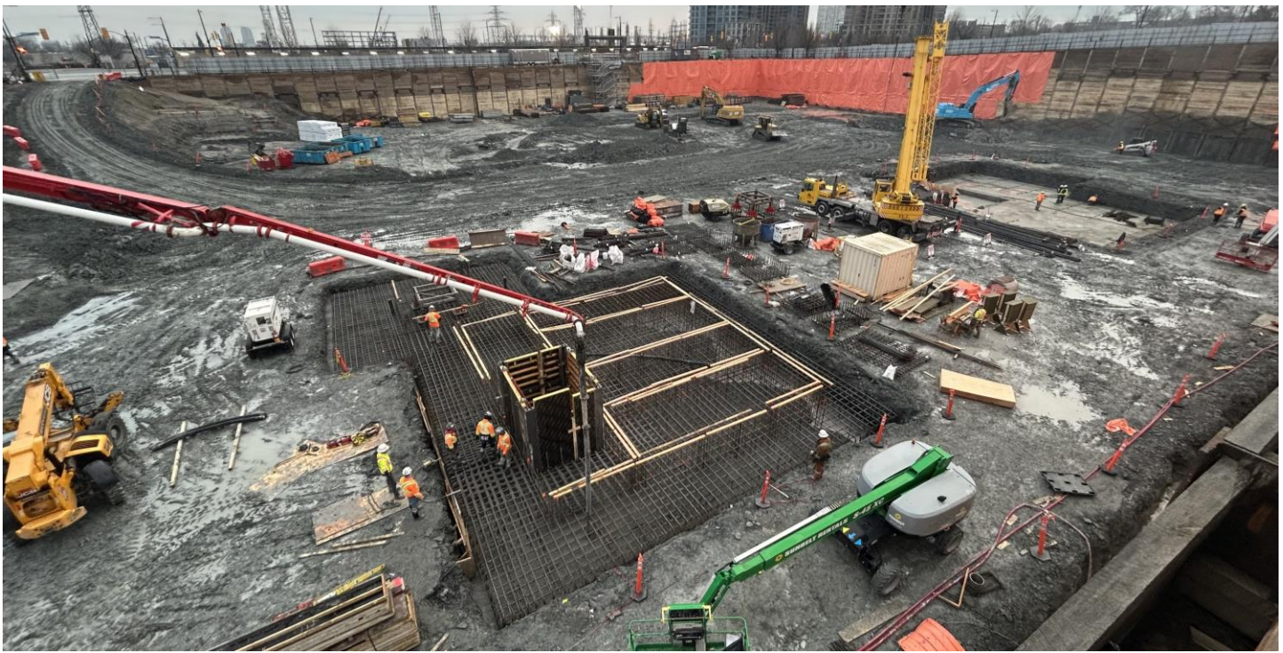
Pictured: Etobicoke Civic Centre progress update as of December 2024.
