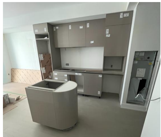
Pictured: Suite Fit-Out Progression.
