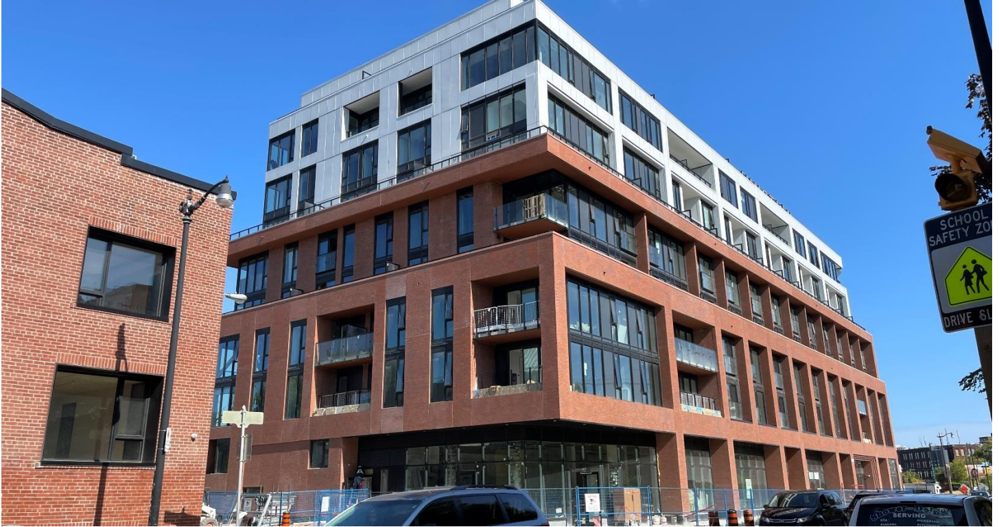
Pictured: Junction House progress update as of October 2023
