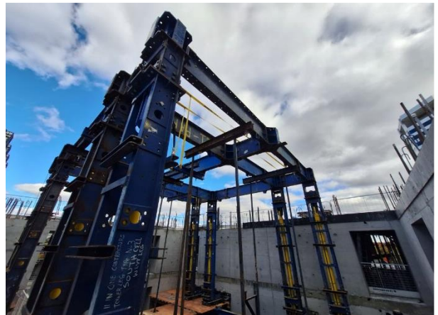
Pictured: Automatic Climbing System (ACS) Installation.
