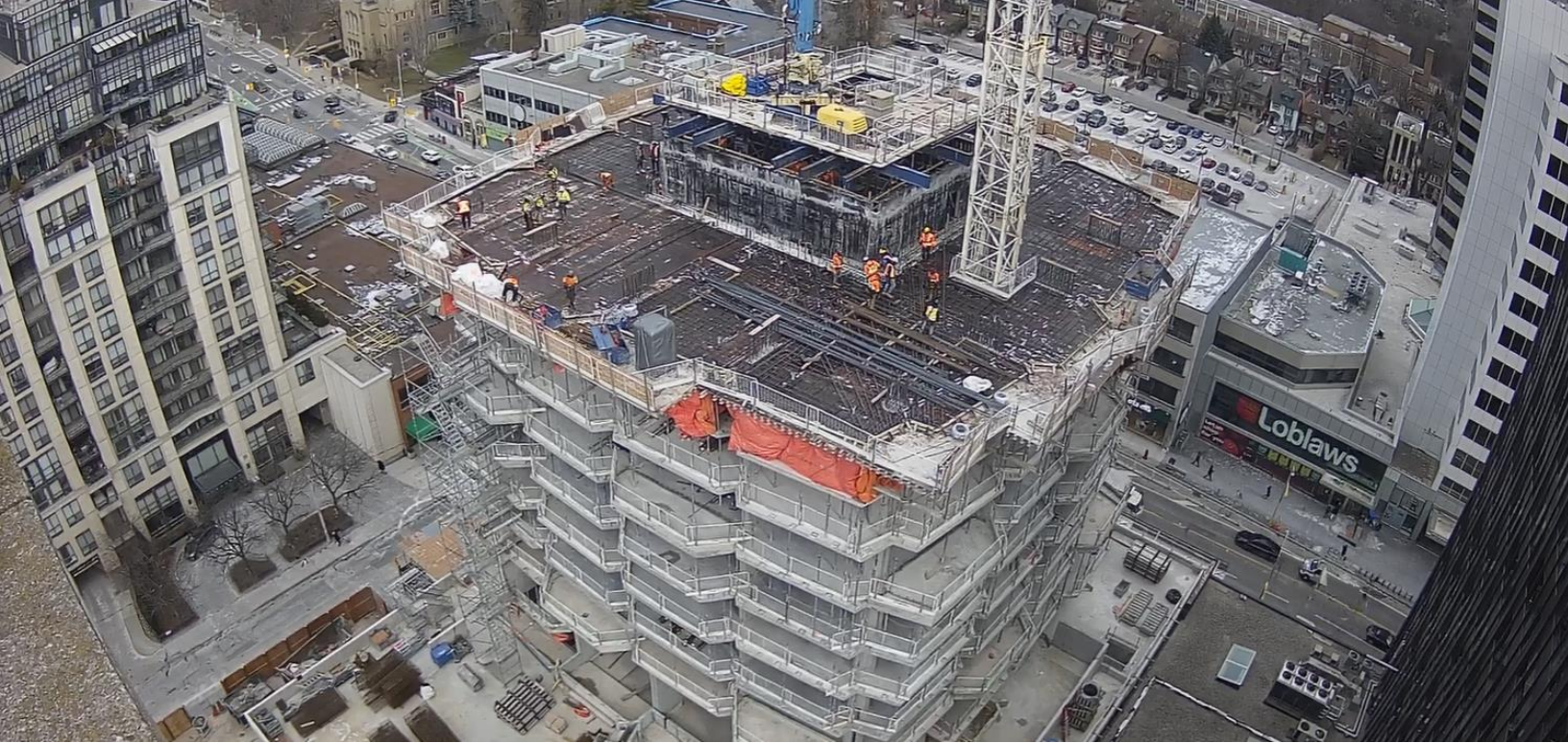
Pictured: One Delisle progress update as of January 2025.
