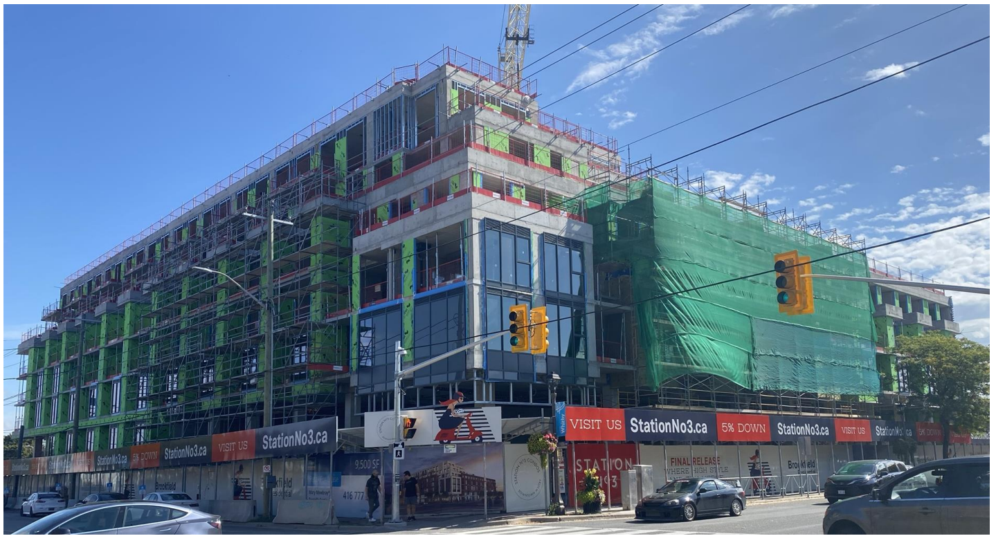
Pictured: Station No.3 progress update as of October 2023
