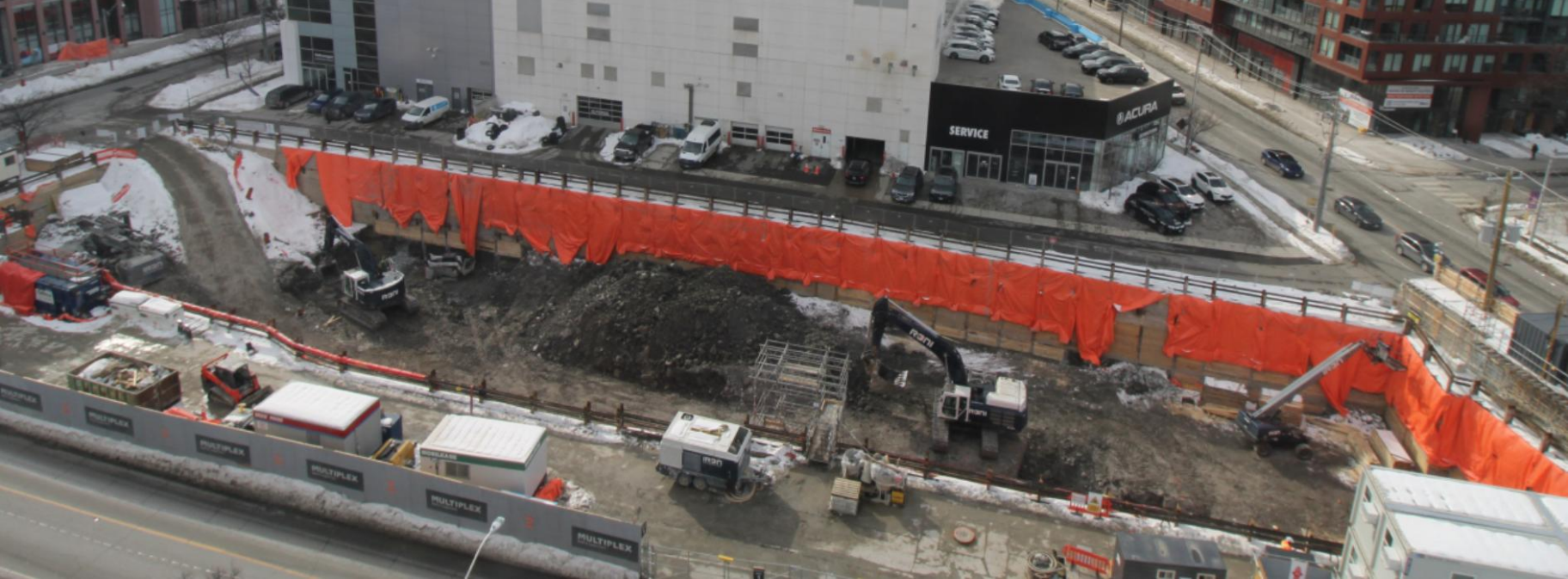
Pictured: Site progress as of February 12, 2026
