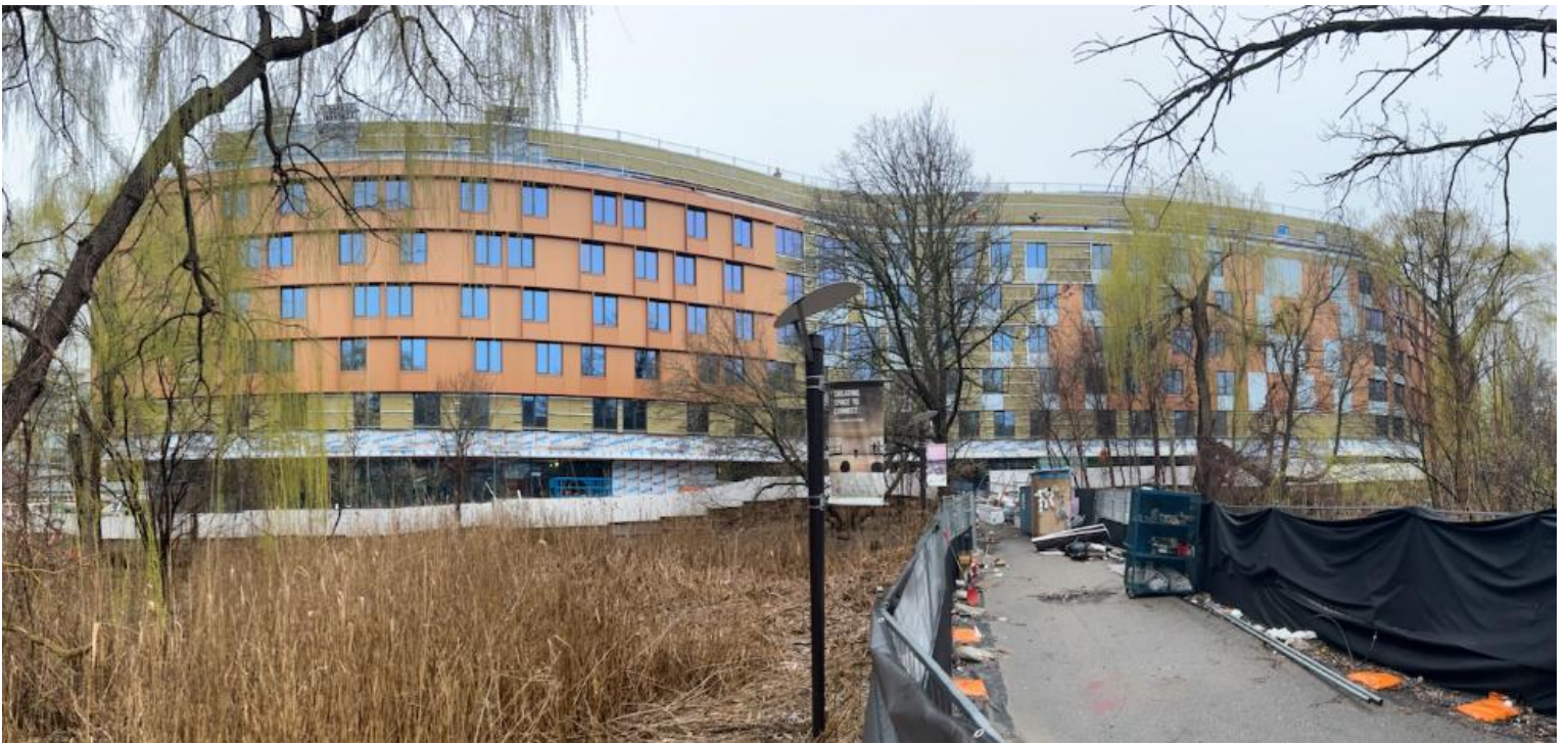
Pictured: Progress update as of April 15, 2026.
