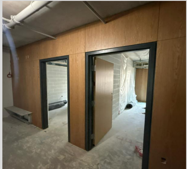
Pictured: Work on the Ground Floor (East).
