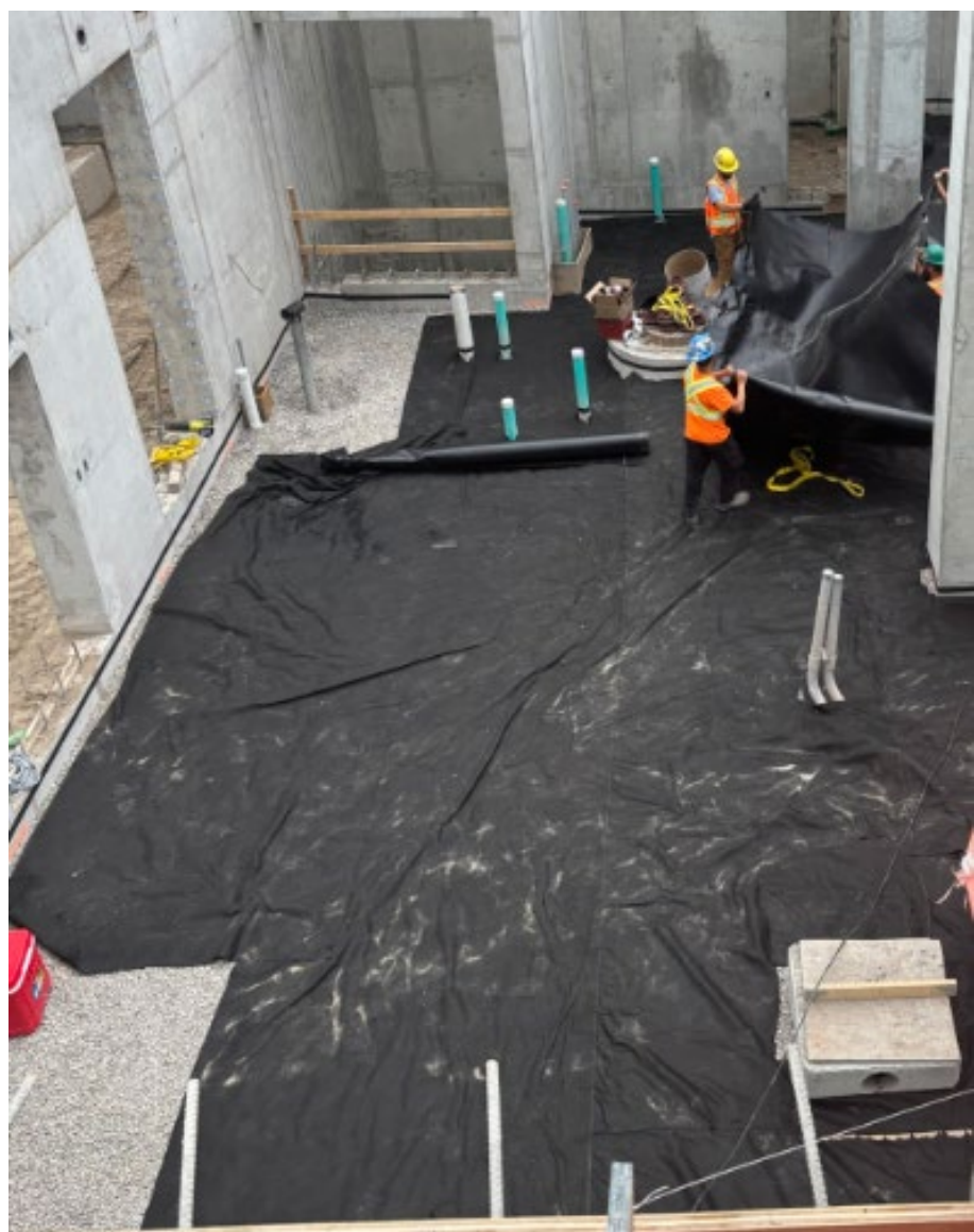
Pictured: Vapour mitigation layer install
