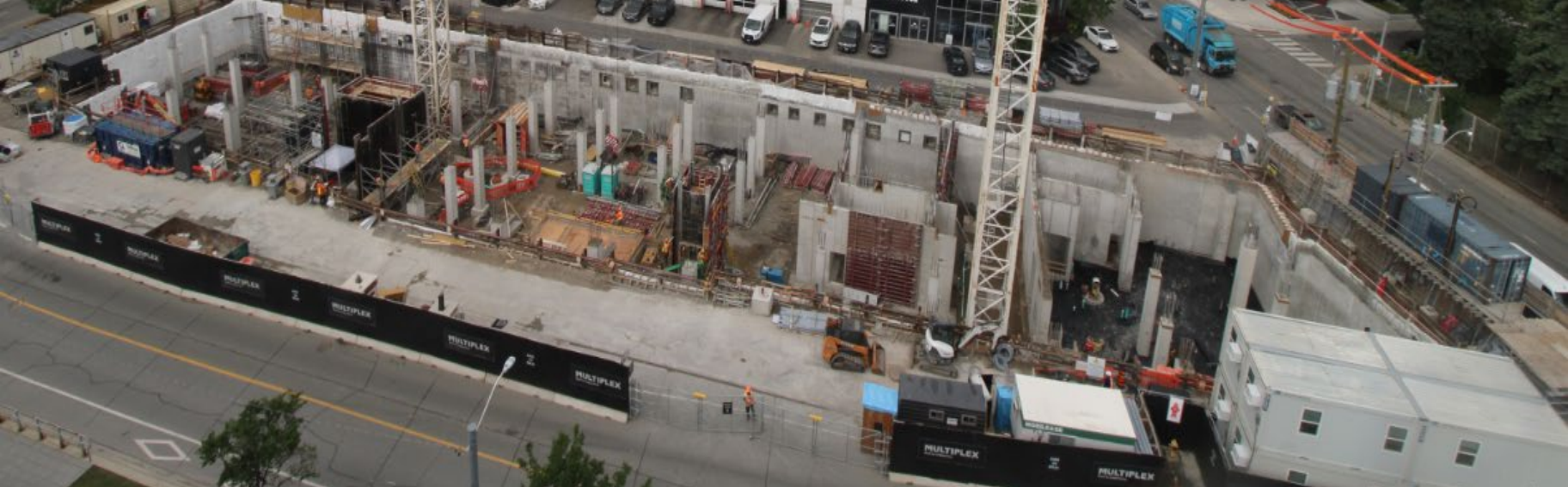
Pictured: Site progress as of June 12, 2026
