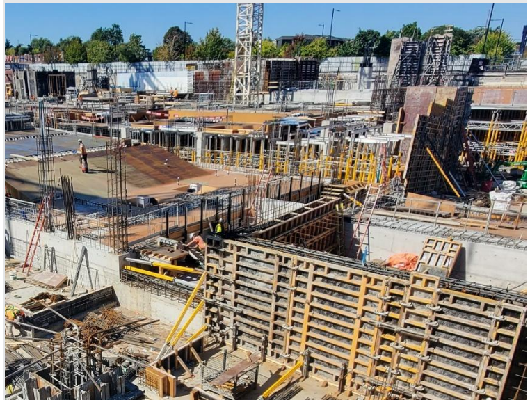
Pictured: The decking of the Level 00 (Ground Floor) concrete slab.
