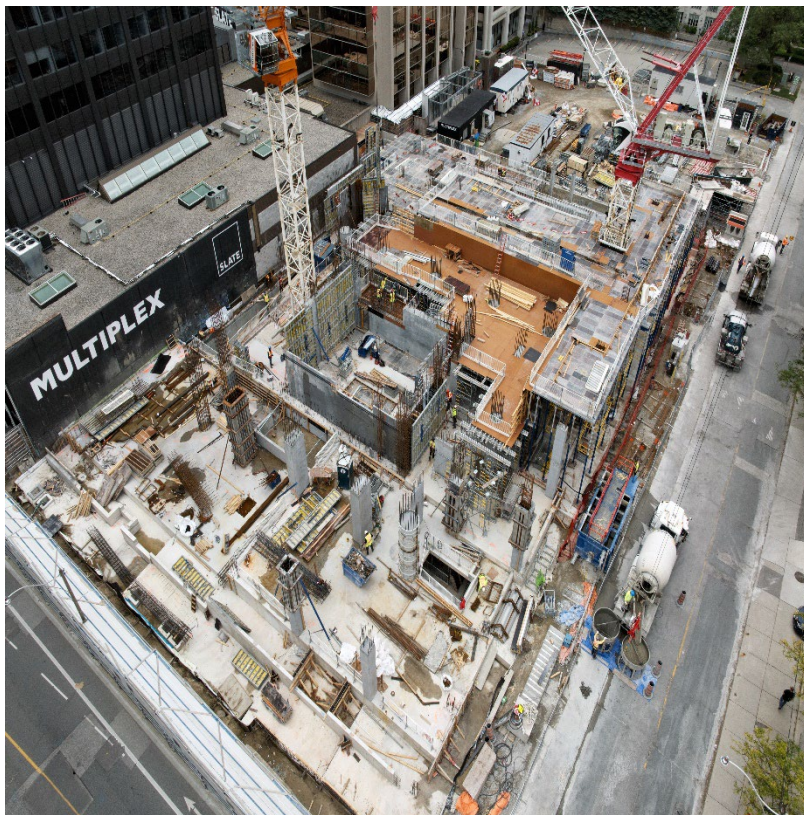
Pictured: One Delisle progress update as of June 2024
