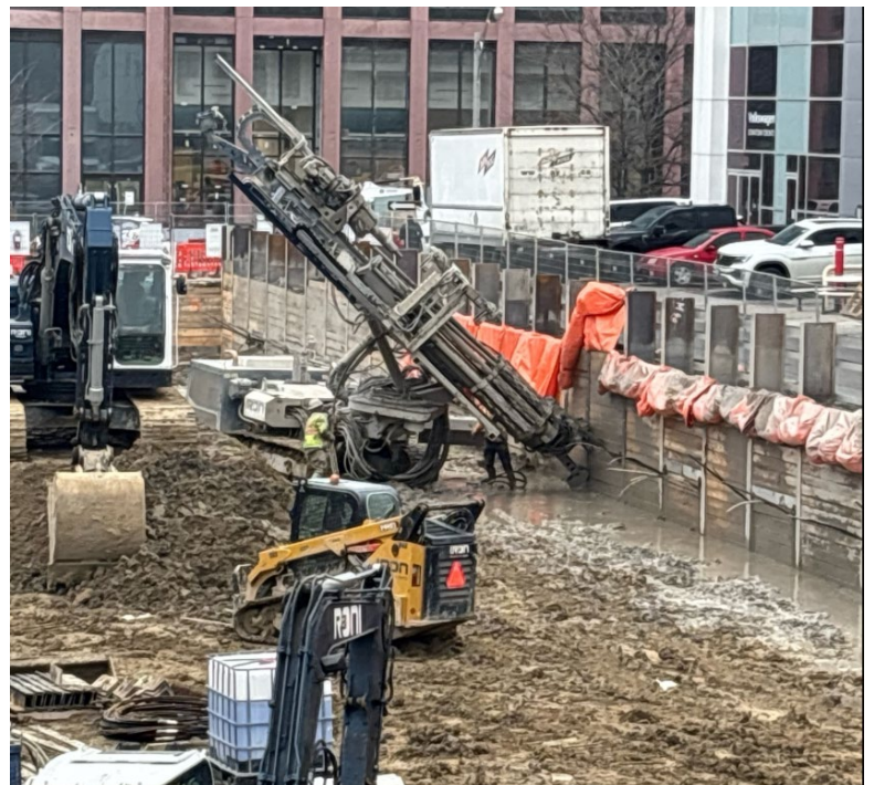
Pictured: Drilling tiebacks on the west elevation
