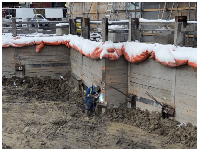
Pictured: welding brackets for tieback stressing on the north wall
