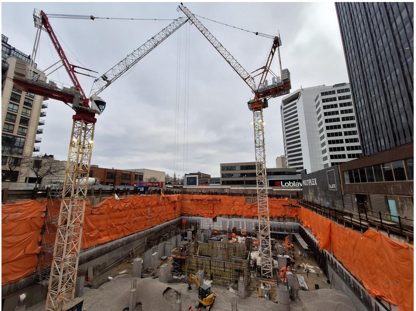
Pictured: One Delisle progress update as of January 2024
