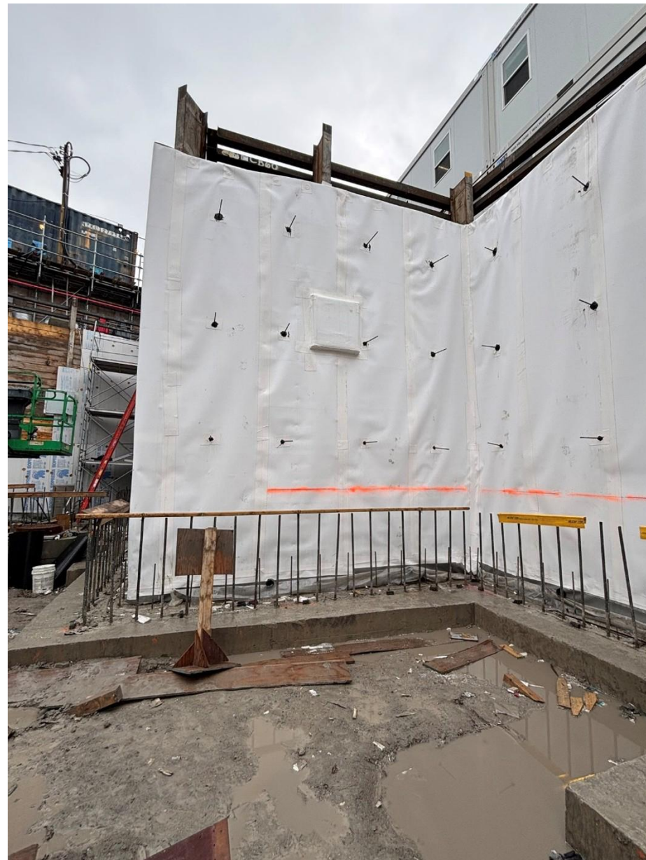
Pictured: Blindside waterproofing install
