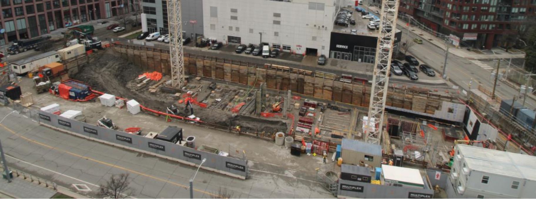
Pictured: Site progress as of April 16, 2026
