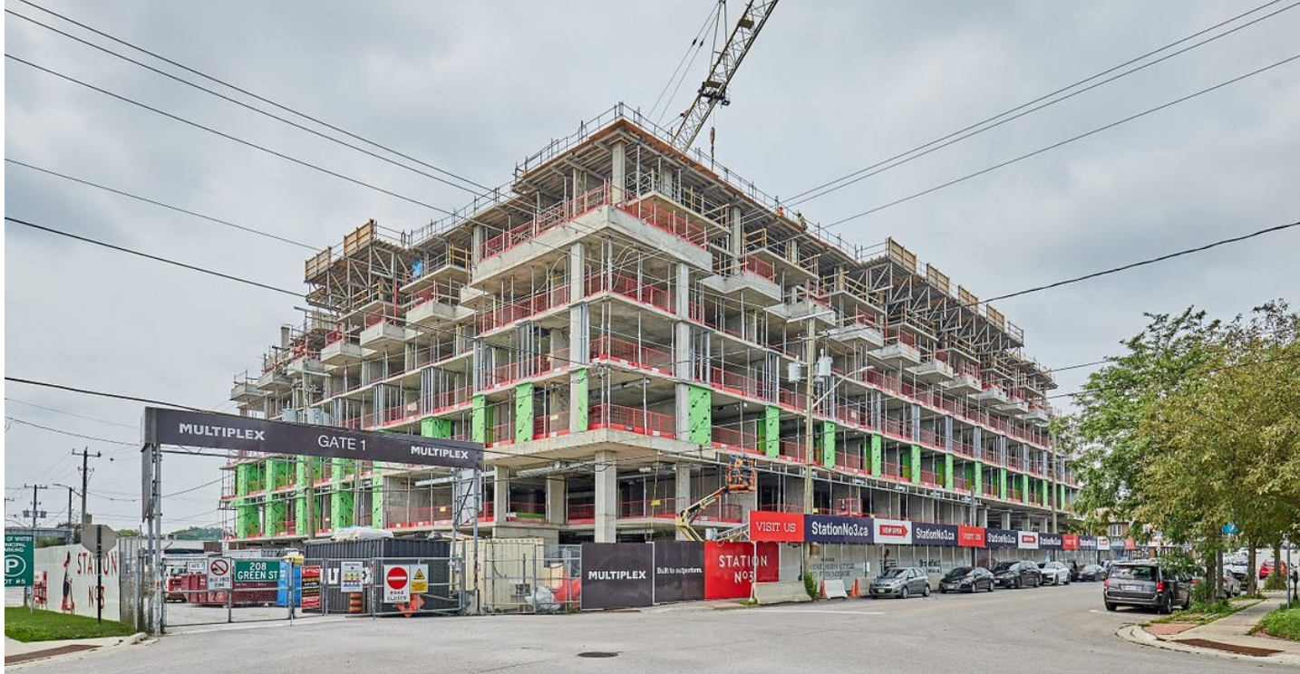
Pictured: Station No.3 progress update as of June 2023
