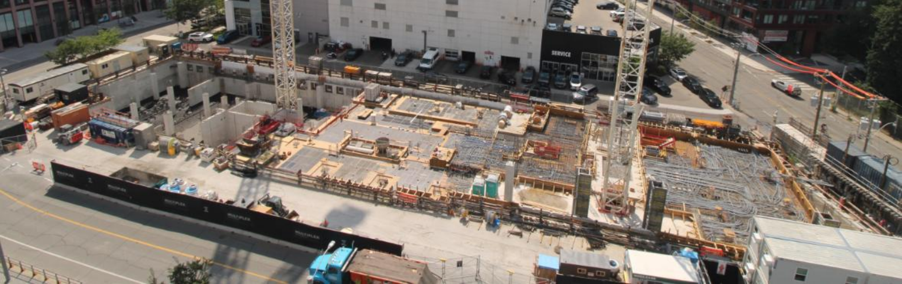
Pictured: Site progress as of August 13, 2026
