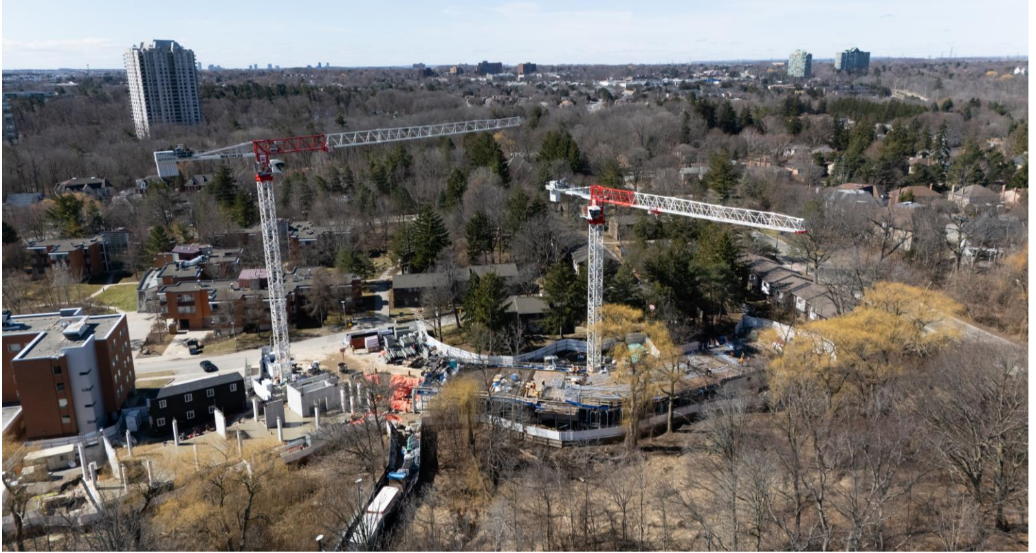
Pictured: Progress update as of March 2025.
