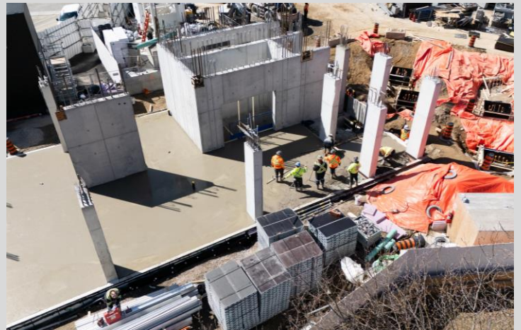
Pictured: Work on slab on grade.
