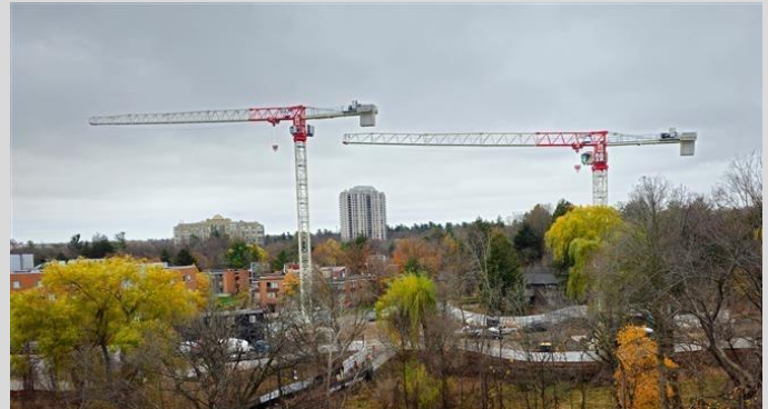
Pictured: Project cranes.
