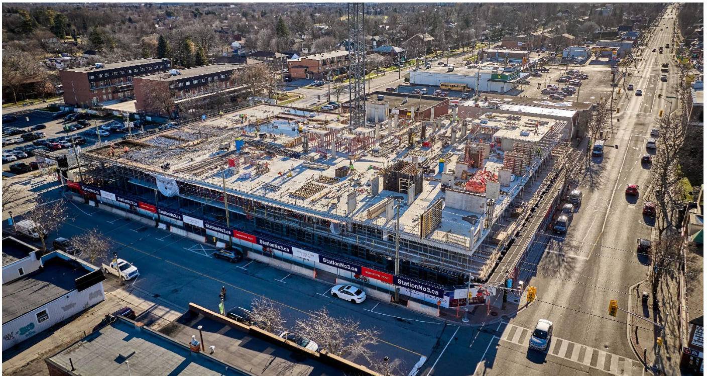
Pictured: Station No.3 progress update as of December
