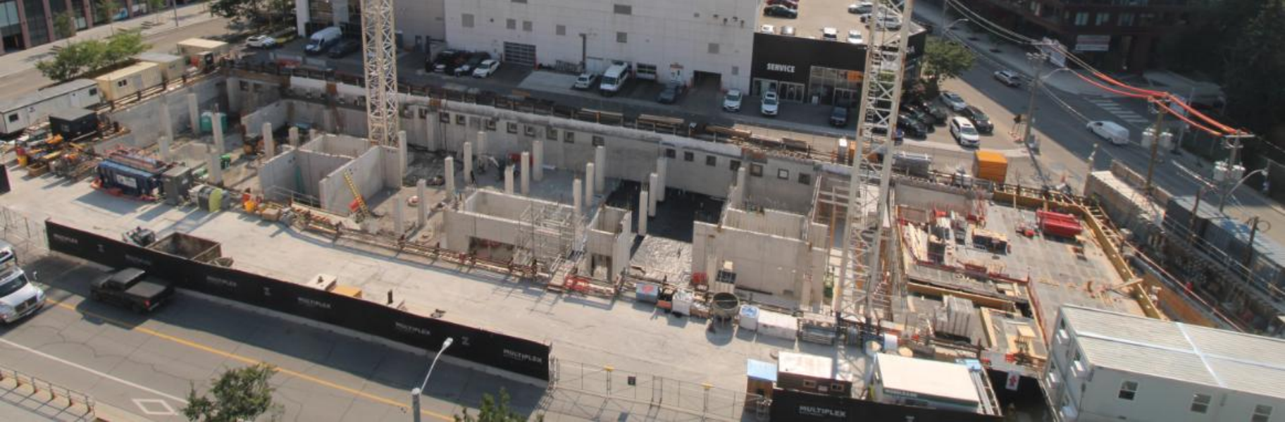
Pictured: Site progress as of July 13, 2026
