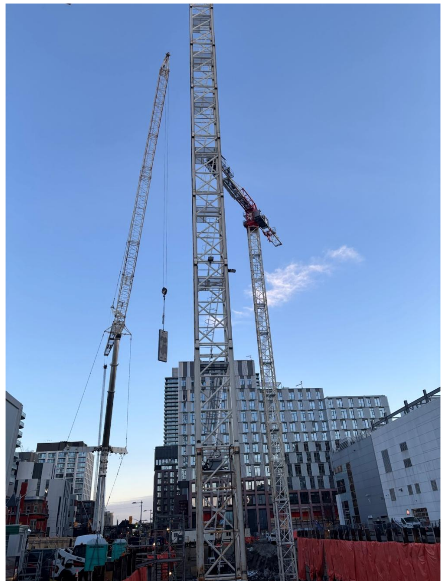
Pictured: Tower crane 2 installation
