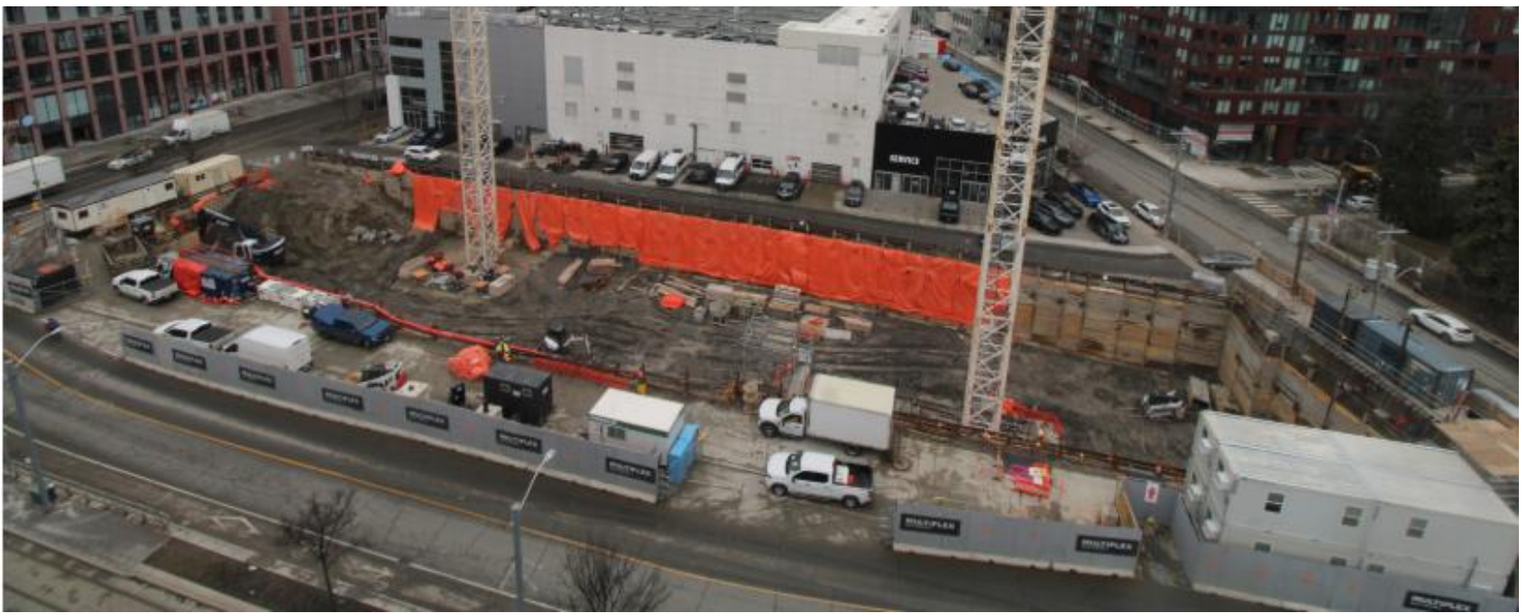
Pictured: Site progress as of March 16, 2026
