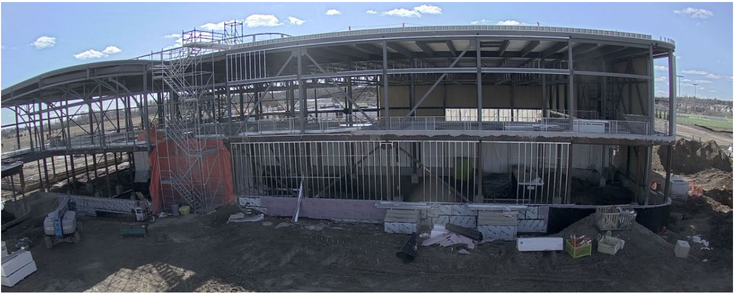
Pictured: Kitchener's indoor recreation complex progress update as of April 1 st 2025.
