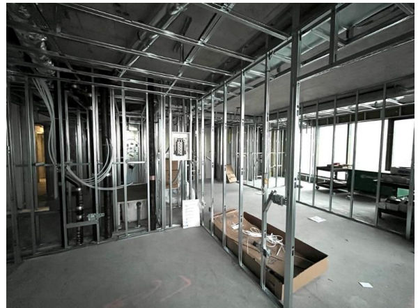
Pictured: Commencement of Interior Suite Framing.
