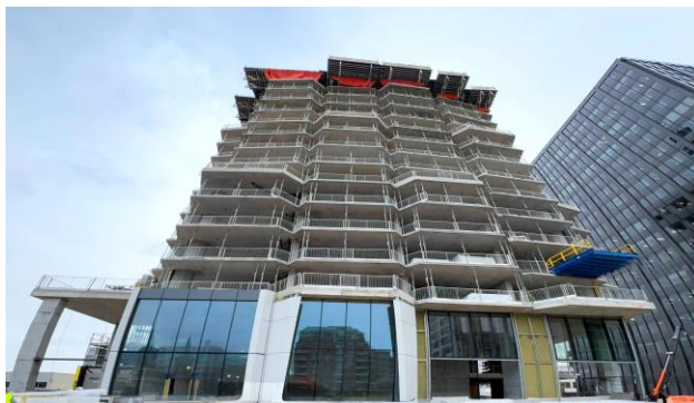
Pictured: Curtain wall installation.
