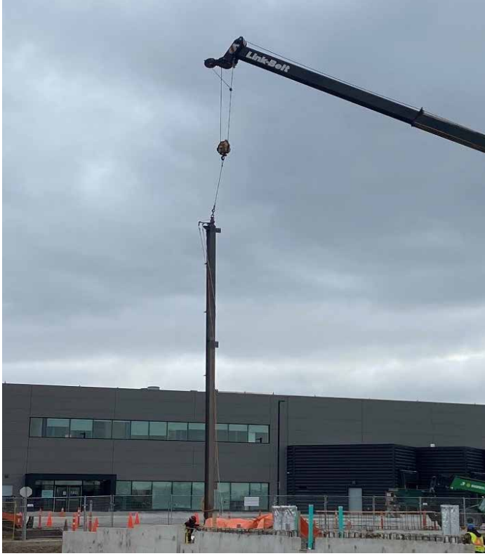
Pictured: OmniaBio B First Steel Column Erection
