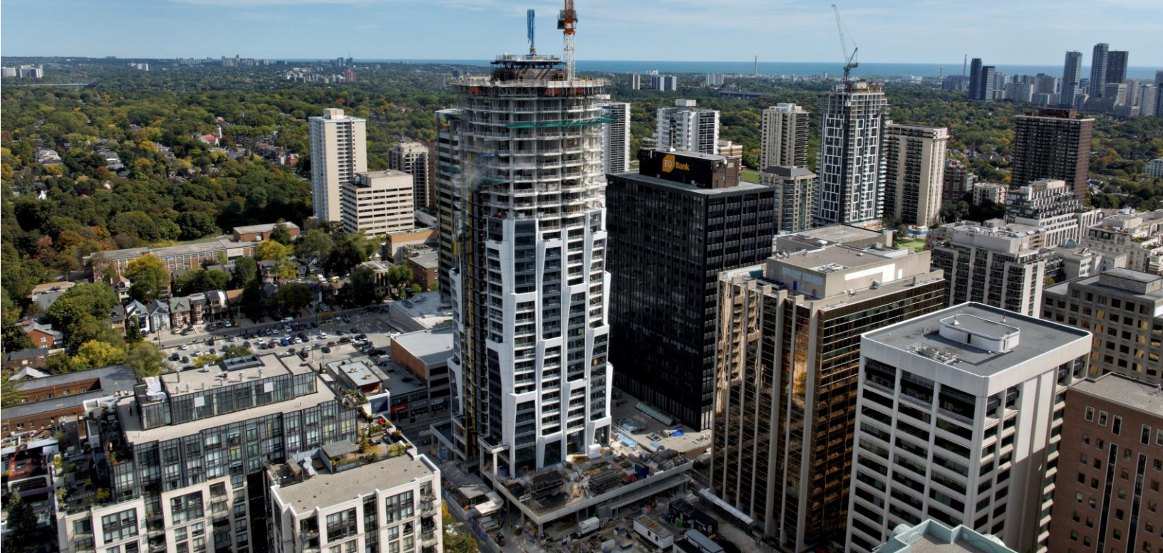
Pictured: One Delisle progress update as of October 2, 2025.
