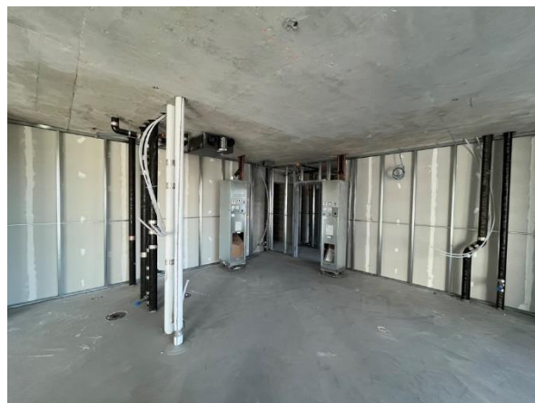
Pictured: Demising Wall Framing
