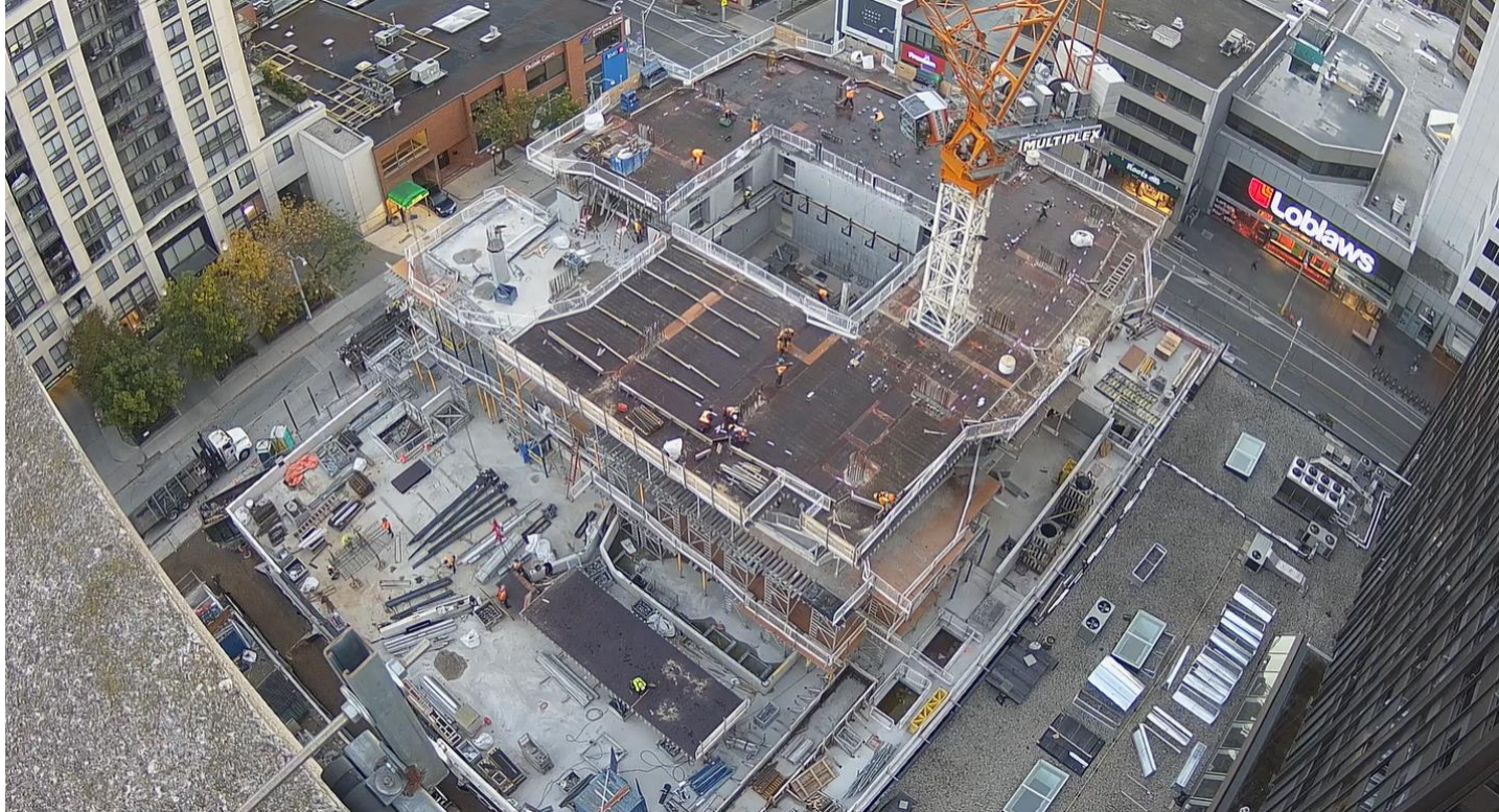
Pictured: One Delisle progress update as of October 2024.
