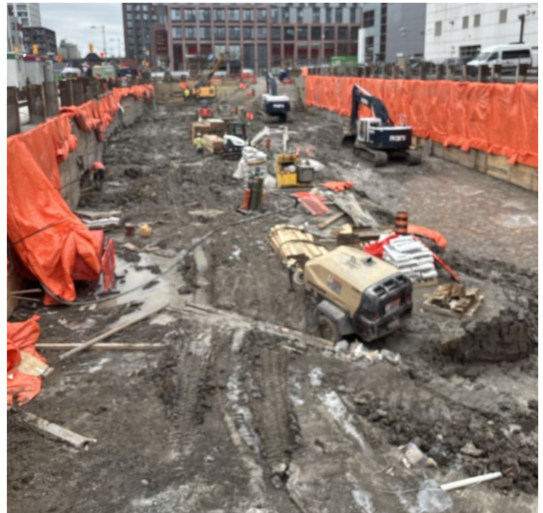
Pictured: Shoring winter protection and conditions
