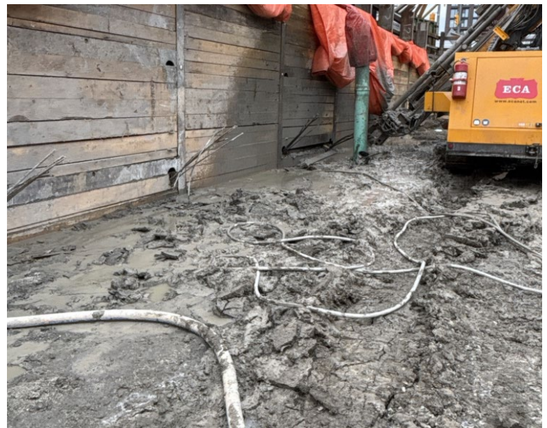
Pictured: tieback install on the east wall
