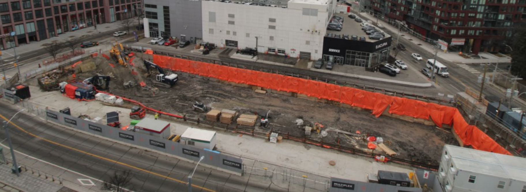
Pictured: Site progress as of January 13, 2026
