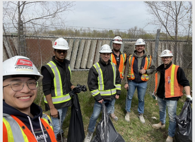
In honour of Earth Day, our dedicated project team at Junction House organized a clean-up collecting litter from public spaces close to Multiplex's construction site.
