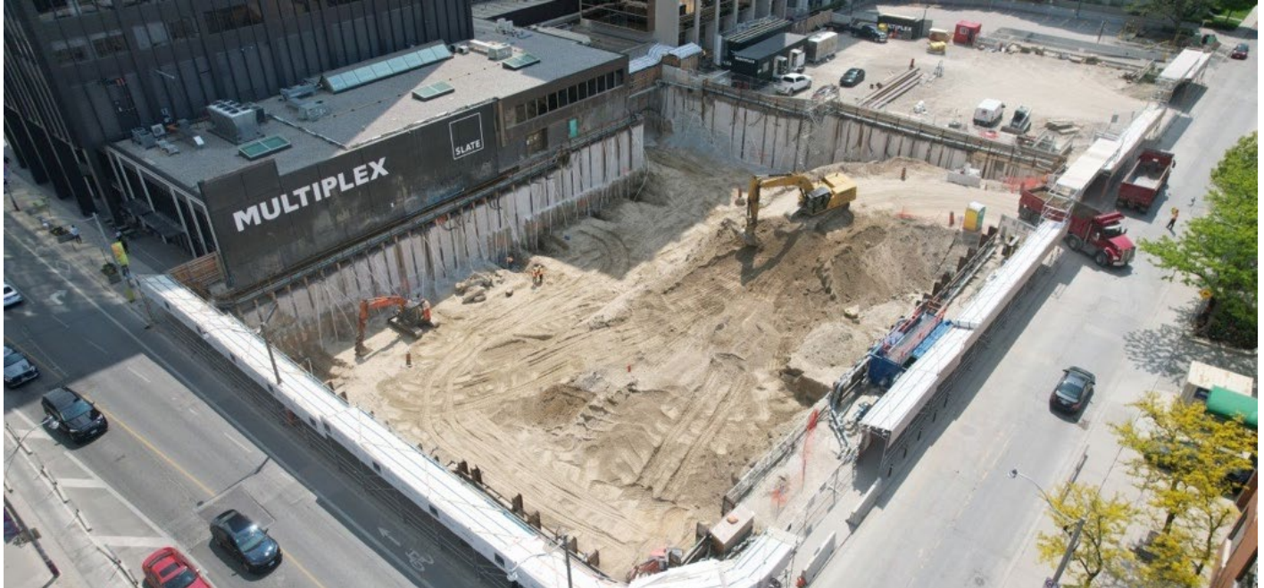
Pictured: One Delisle progress update as of June 2023
