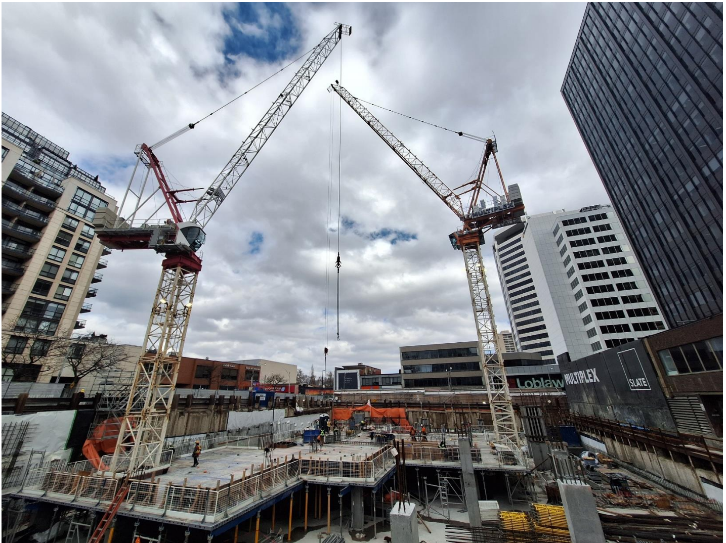
Pictured: One Delisle progress update as of March 2024
