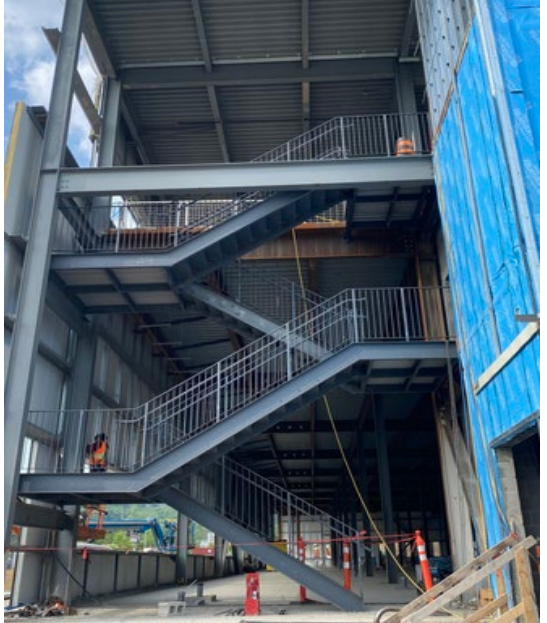
Pictured: OmniaBio B Stair 1 at North-East corner
