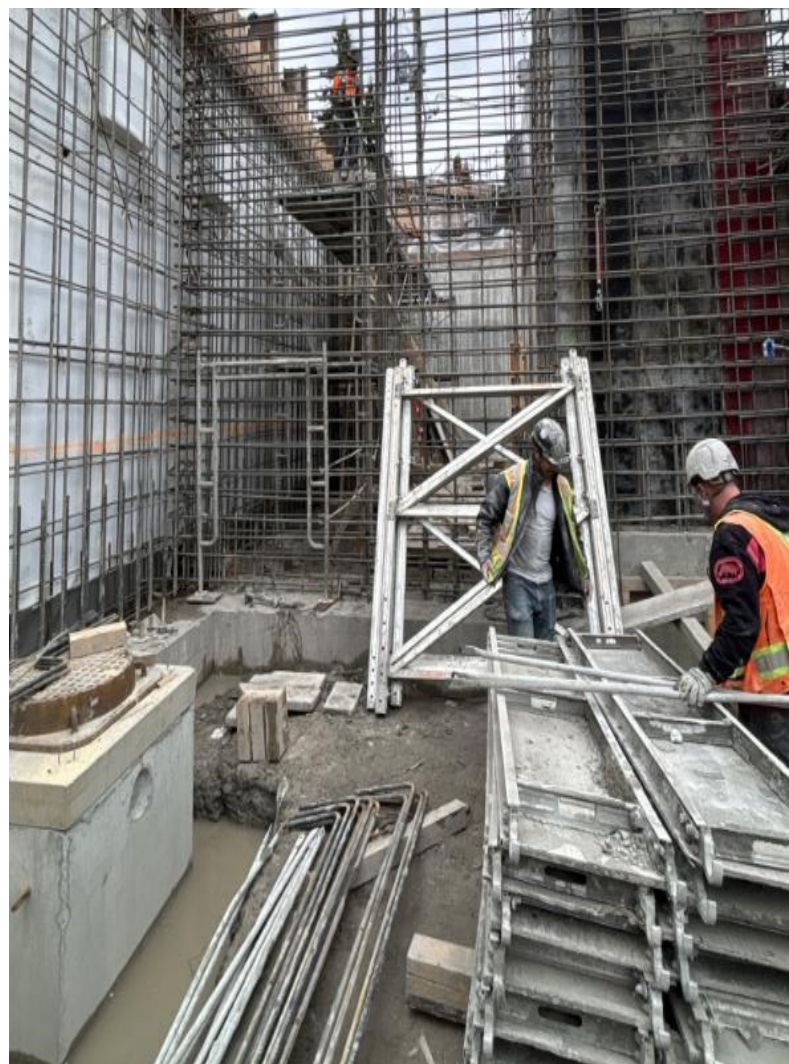
Pictured: internal wall rebar install
